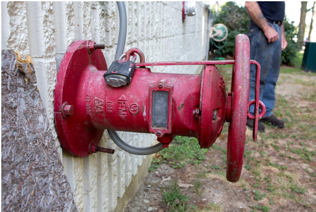
System 1 - East Side of Building
