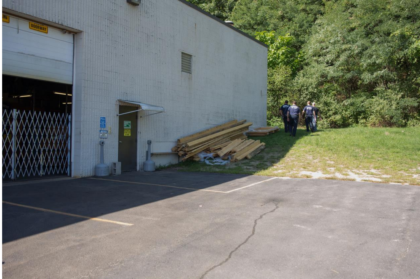
North Side - Egress Door
